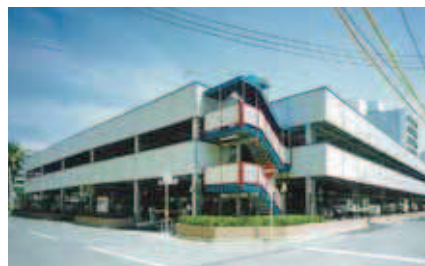
City Parking Hakata Station East (Fukuoka)
