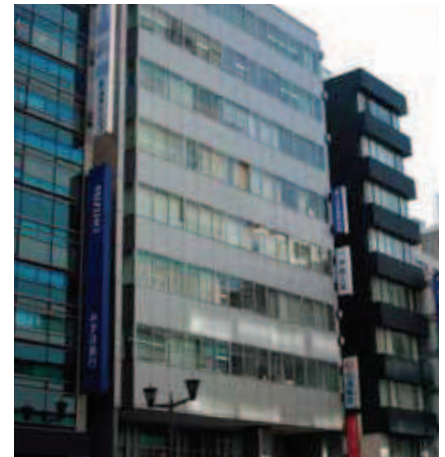
Yanagiya Taiyo Building (Tokyo)
