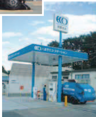
Natural Gas Eco Station (Hachioji)
