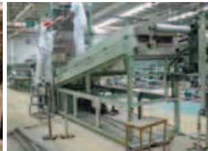
Equipment disassembly and installation
